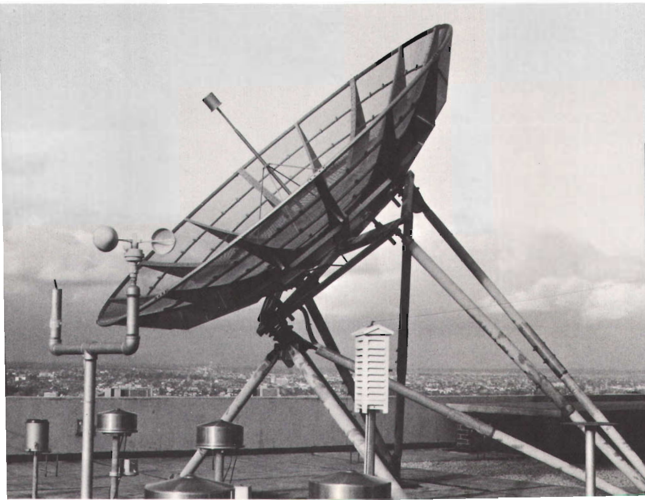
(Below) Signals from the Japanese Geostationary Meteorological Satellite are received by a 5 metre diameter dish antenna located on the roof of the Bureau of Meteorology building in Melbourne. Pictures are received every three hours, and in addition to routine forecasting, are used for locating and tracking cyclones and other severe weather events.
